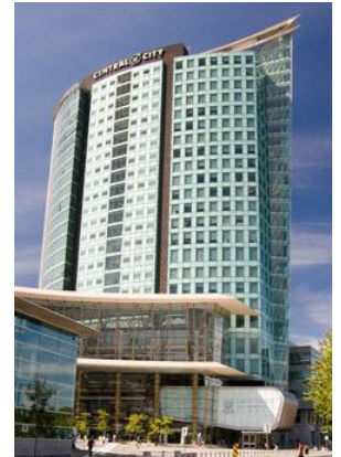
McQuarrie Hunter’s new offices
